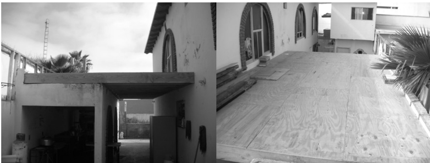
Floor for the new addition to the ministry center
